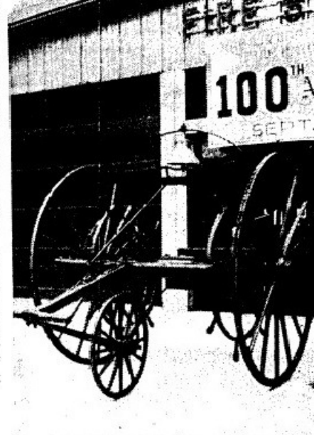
HR GRACE—Hose reel is part of original equipment dating back to 1863. Hydrants were installed in 1863.
